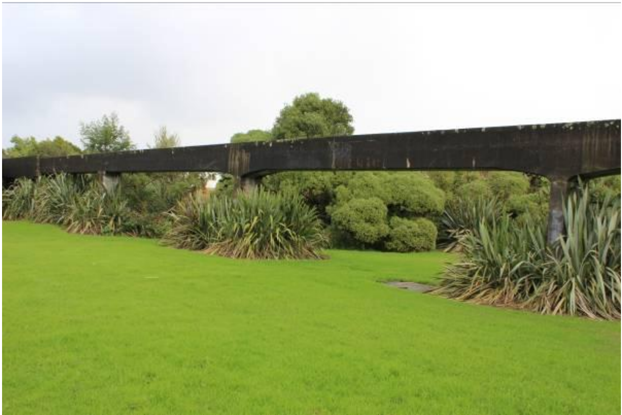
Flax under Sewer
